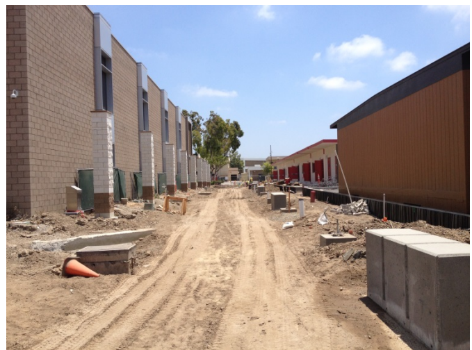
CMU pilasters, light pole bases, and concrete benches at the north pedestrian walkway.
