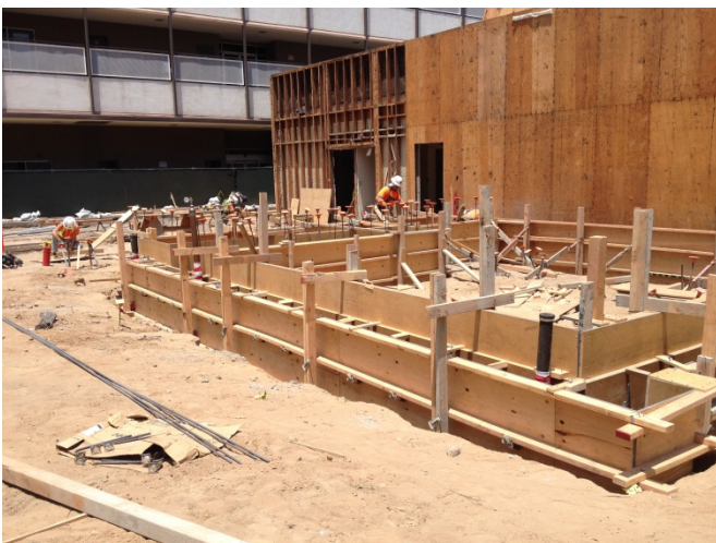
Stem walls formed and ready for concrete pour.
