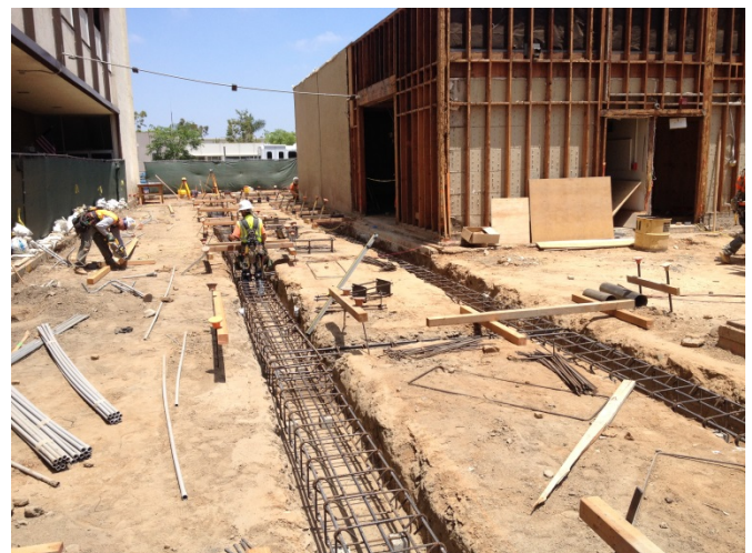
Rebar cages for covered walkway footings around north and west sides of Planetarium building.
