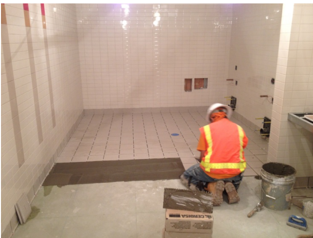
Restroom tile installation in progress.
