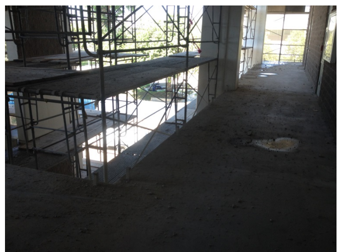
Guardrail demolition completed.
