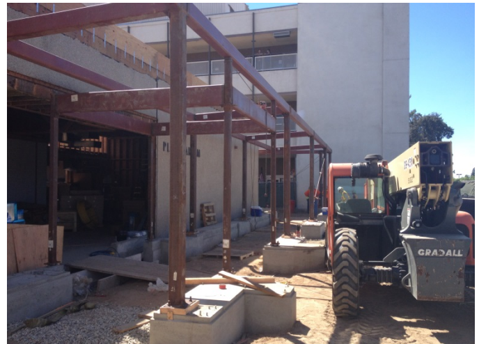
Welding activities ongoing for the covered walkway structural steel frame.
