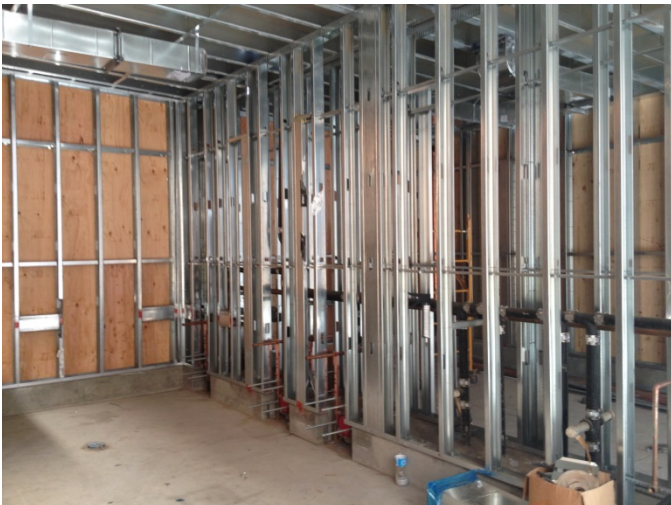
Steel stud framing completed. Plumbing rough-in ongoing.
