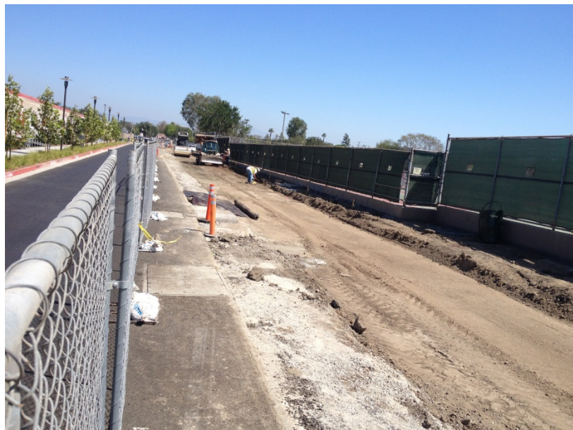
Fine grading south side of Campus Road.
