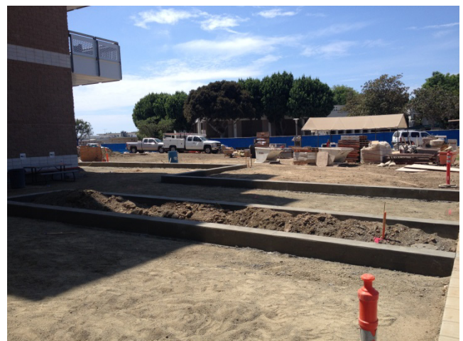
Concrete border poured around future walkways to Dunlap Hall.
