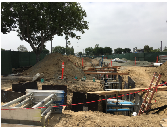
Installation of chilled water pipe at Parking Lot 6
