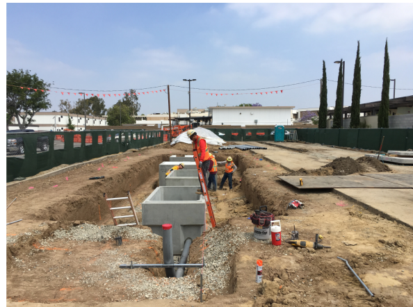
Installation of vaults and conduit at Electrical Building
