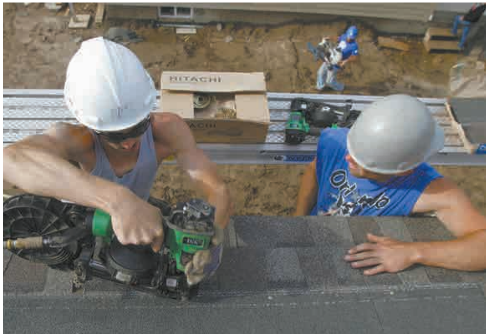
Zach Schmiesser, of West Des Moines, Iowa, left, and Dustin Zuck, of Des Moines, shingle a home in Des Moines. Students enrolled in the Des Moines Area Community College construction program have spent the last several weeks constructing new homes Des Moines.
