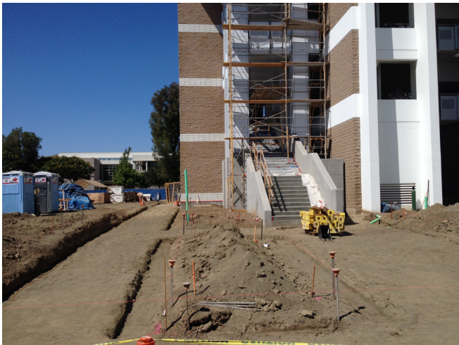
Grading for unit pavers and concrete bands.
