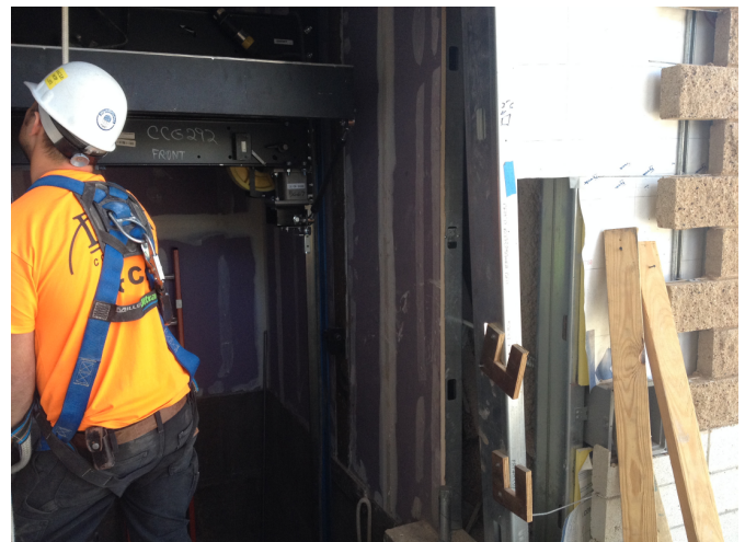
Guiderails being installed in new elevators.
