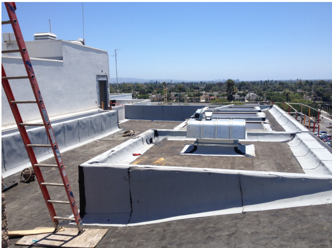
Built-up roofing being installed on new addition roof.
