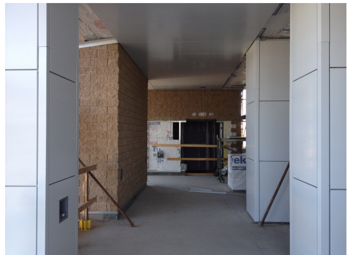
CMU veneer installed and Centria panels being installed on new addition columns and ceilings.
