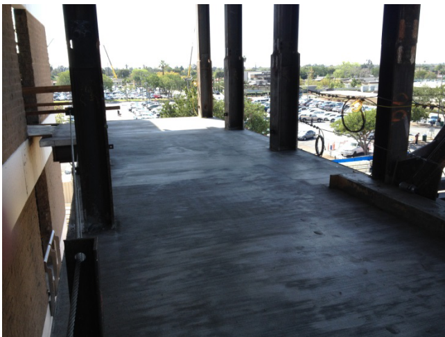
Concrete decks poured at new elevator addition.
