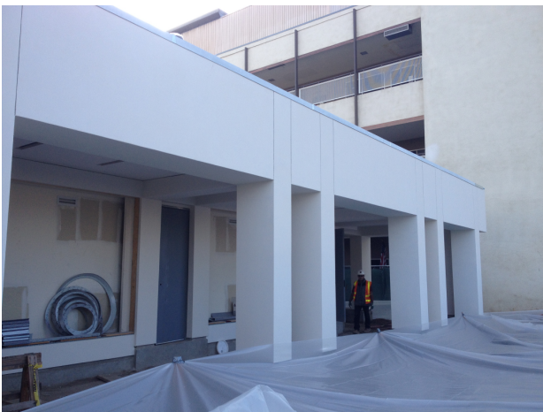
Exterior plastering completed.
