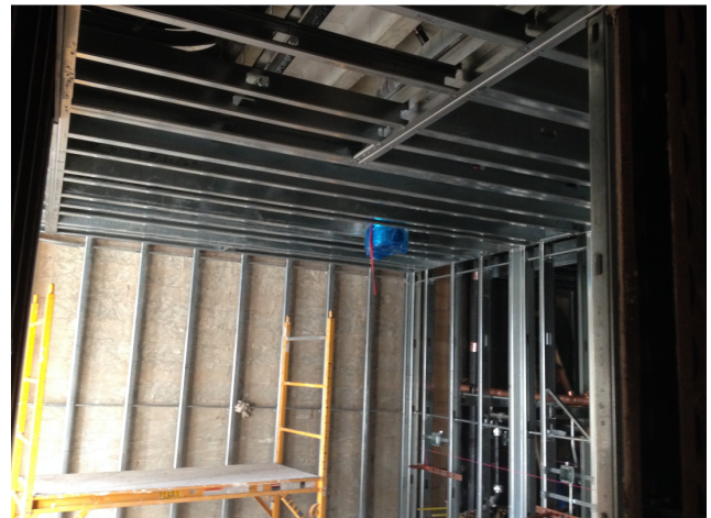
Steed stud framing activities at second floor restroom.
