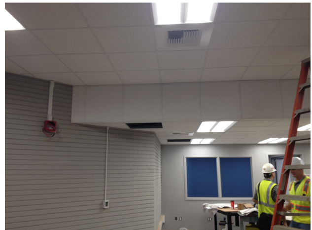
Ceiling tile and light fixtures installed.
