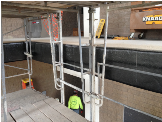
Fiber wrap installed on deck edges.
