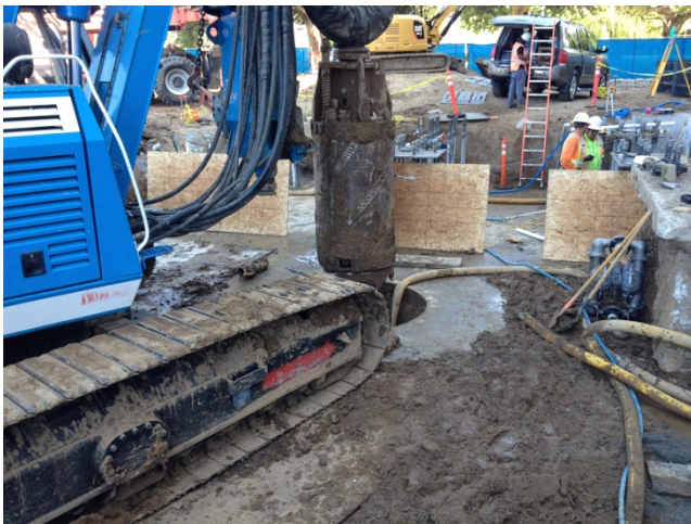
Drilling rig removing soil from the bottom of the drilled hole.
