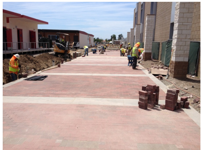
Pavers, concrete bands, and landscaping being installed at north pedestrian walkway.
