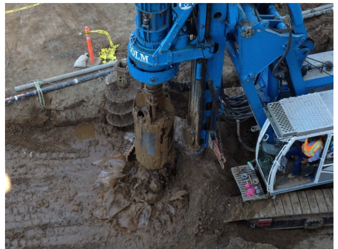
Overhead view of drilling rig dumping soil from core barrel.
