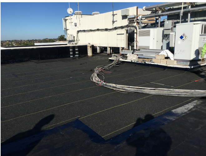
Capsheet being installed on south side of roof.
