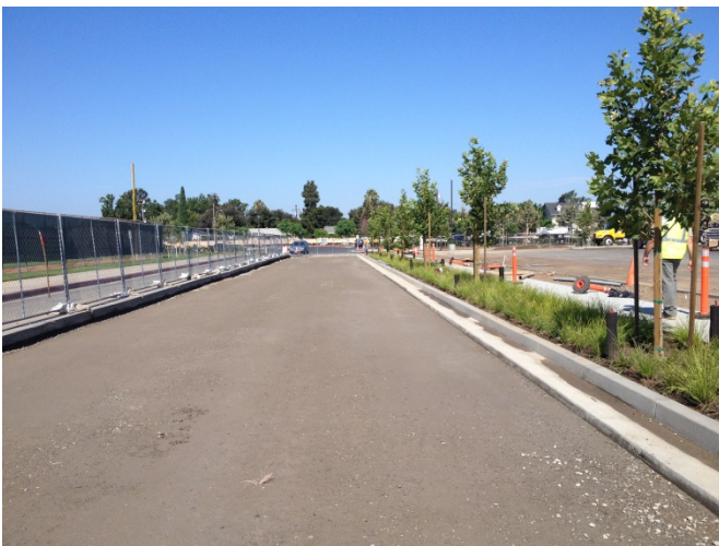
North side of Campus Road ready for AC paving.
