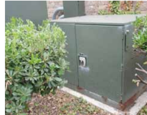
Typical Pad Mount 15KV Selector Switch
