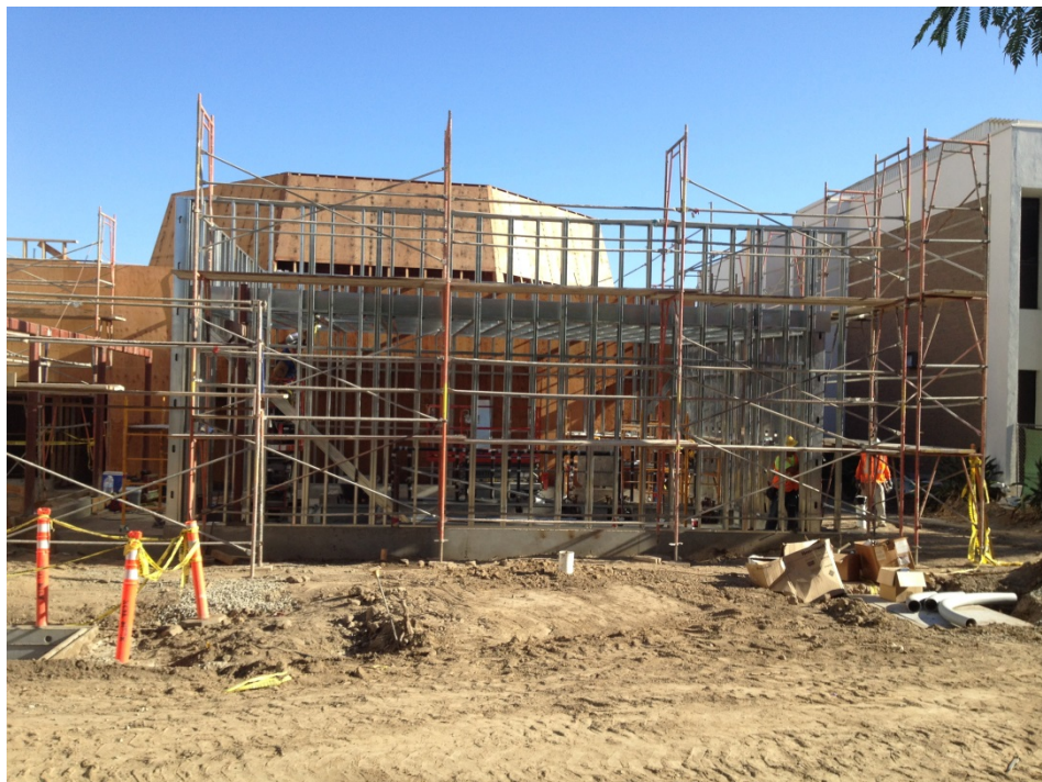
Scaffold erected and steel stud framing ongoing at restroom addition.
