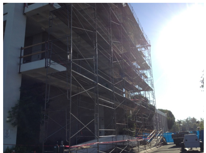
Scaffold up and guard rails being removed from 2 nd , 3 rd , and 4 th floors.
