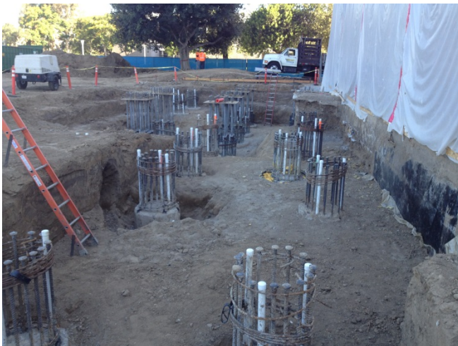
Piles completed where future elevators will be constructed.
