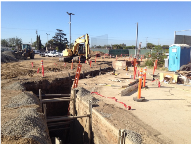
Storm drain tie-in to newly completed retention basin.
