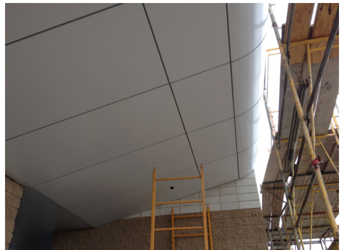
Centria panels installed on 4 th floor new addition ceiling.
