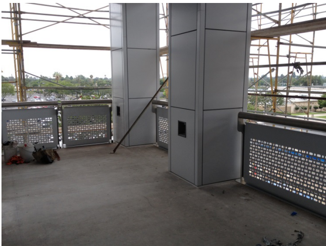
Stainless steel guardrails and infill panels installed on all levels of new addition.
