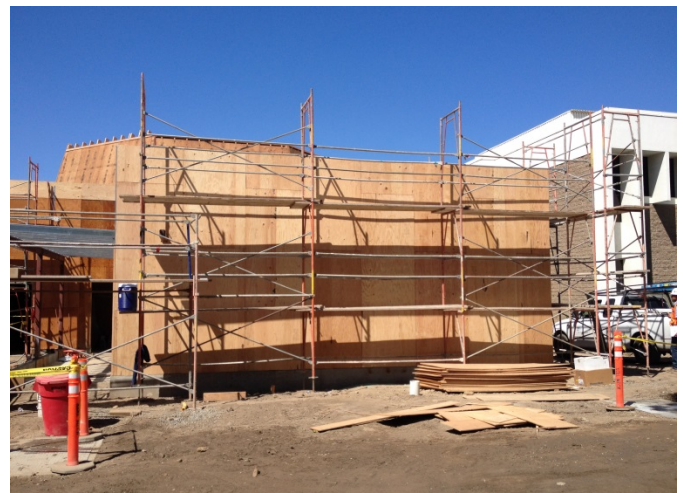
Wall sheathing installed around restroom addition.
