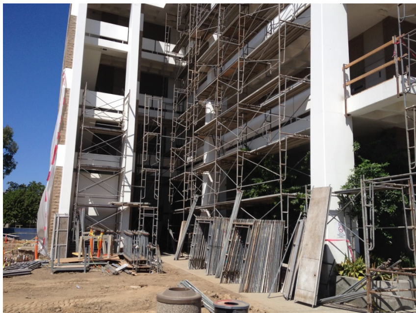
Last remaining scaffold being erected around the building.
