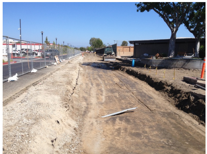
Over excavation and compaction operations on south side of Campus Road.
