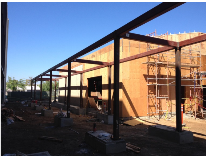
Structural steel erected for the covered walkway.
