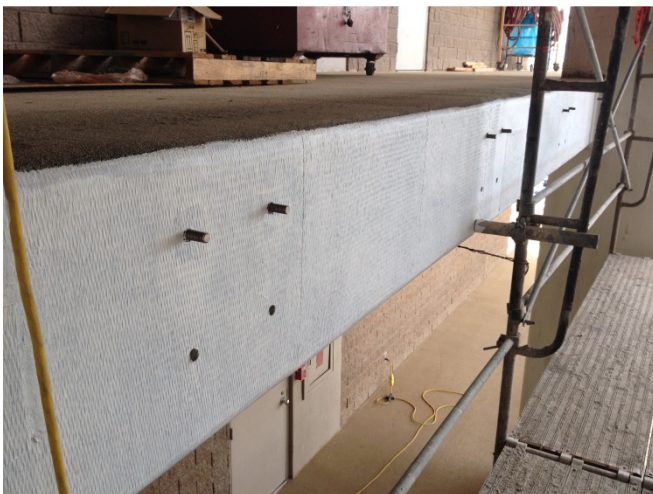
Vertical faces of balconies being painted and anchors for stainless steel guardrails being installed.
