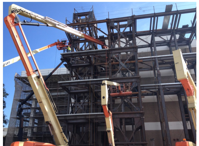
Welding activities on structural steel.
