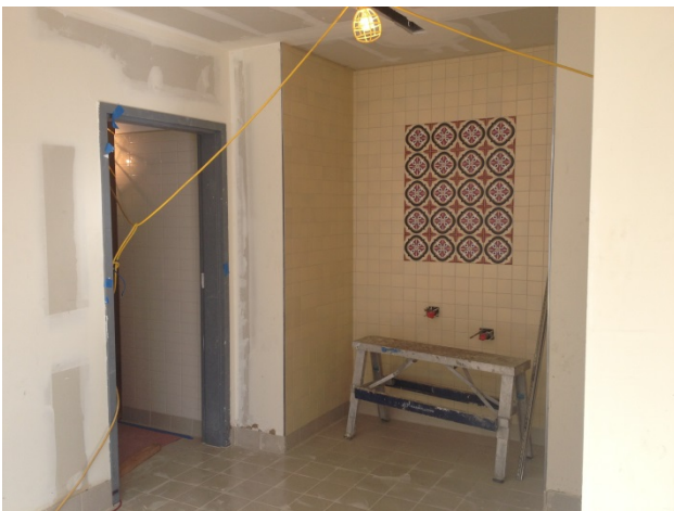
Tile install ongoing at restroom addition vestibule.
