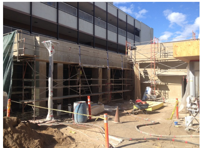
Covered walkway scratch and brown coating being applied.
