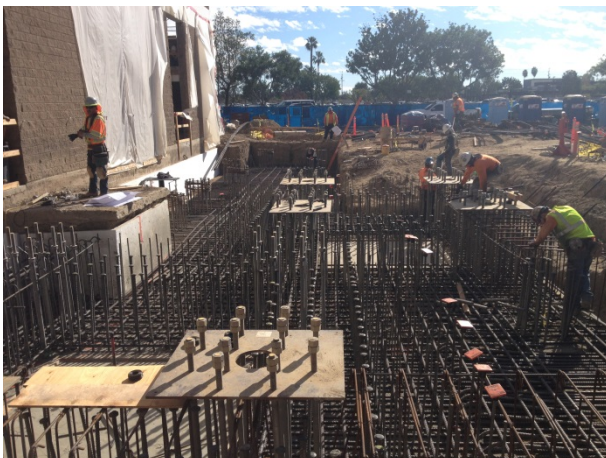
Pile cap rebar being placed at new elevator pit, prep for 300 CY concrete pour.
