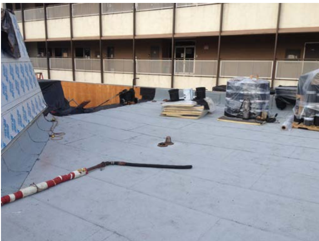
Install of built-up roofing on main roof ongoing.
