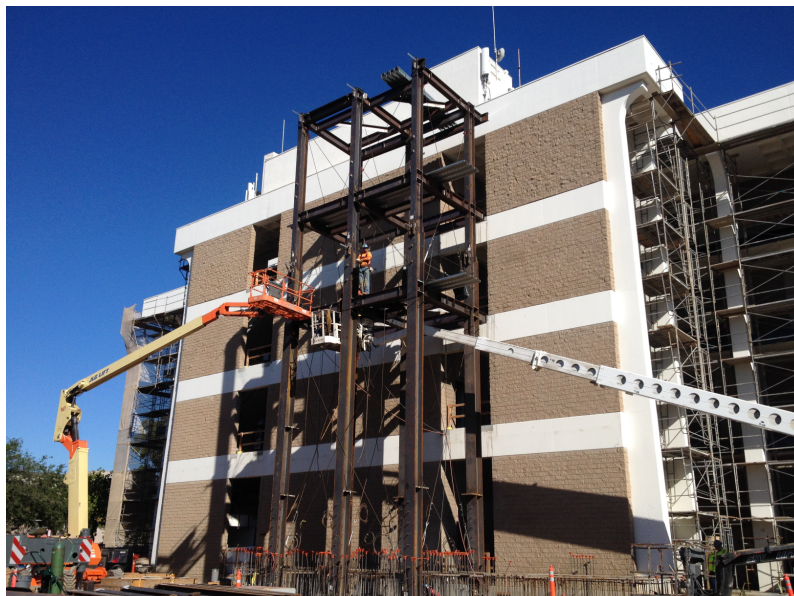
Plumb-up, bolt-up, and welding activities on structural steel addition.
