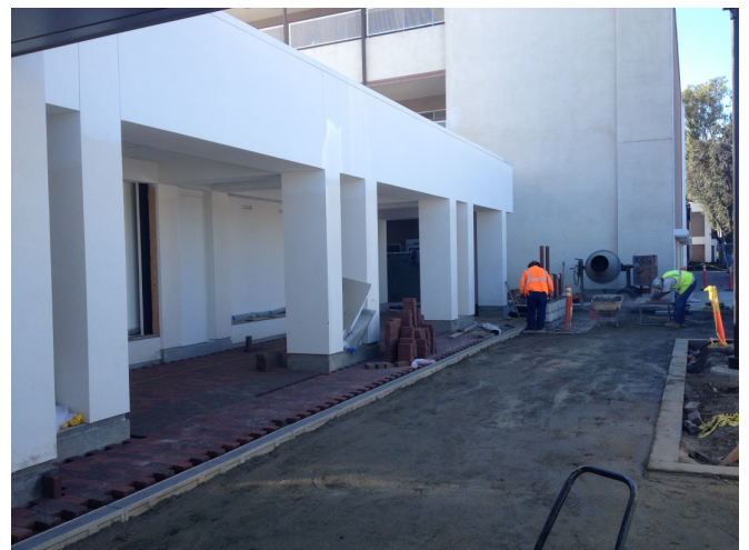
Pavers being installed under canopy, CMU platform for monument sign being constructed.
