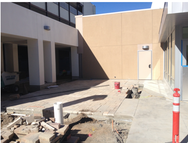
Decorative pavers being installed south side of Planetarium.
